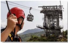
Cable car maintenance
