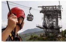
Cable car maintenance
