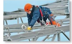
Work at height
