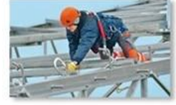
Work at height
