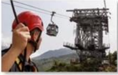
Cable car maintenance
