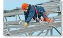
Work at height
