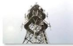
Mobile plant maintenance
