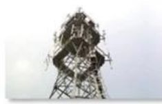
Mobile plant maintenance
