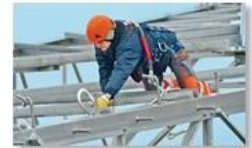
Work at height
