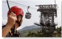
Cable car maintenance
