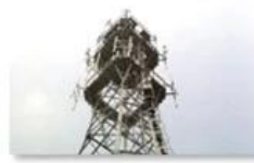
Mobile plant maintenance
