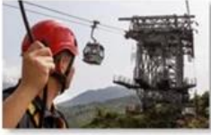
Cable car maintenance
