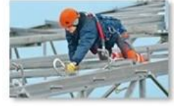
Work at height
