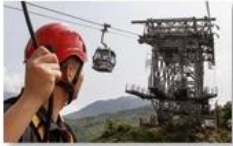
Cable car maintenance
