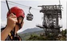
Cable car maintenance
