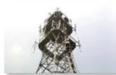
Mobile plant maintenance
