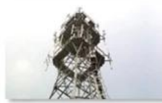
Mobile plant maintenance
