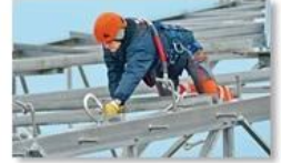
Work at height
