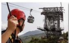
Cable car maintenance
