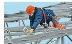
Work at height
