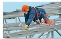
Work at height
