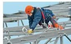
Work at height
