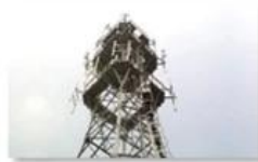
Mobile plant maintenance
