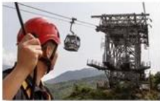
Cable car maintenance
