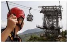
Cable car maintenance
