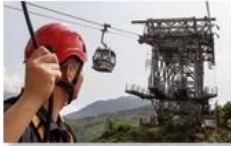
Cable car maintenance
