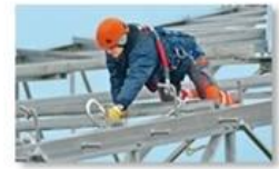
Work at height
