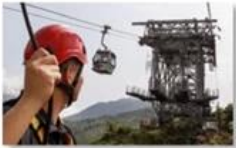
Cable car maintenance
