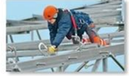
Work at height
