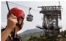
Cable car maintenance
