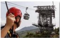
Cable car maintenance
