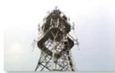
Mobile plant maintenance
