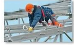
Work at height
