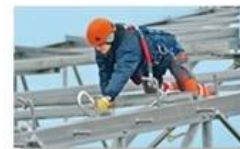
Work at height
