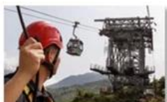
Cable car maintenance
