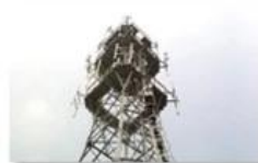
Mobile plant maintenance
