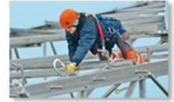
Work at height
