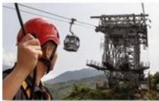
Cable car maintenance
