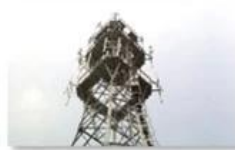
Mobile plant maintenance
