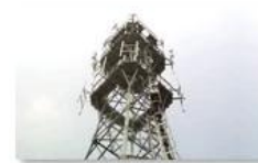
Mobile plant maintenance
