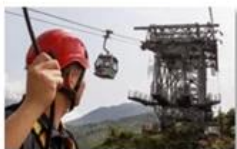
Cable car maintenance
