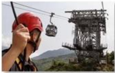
Cable car maintenance
