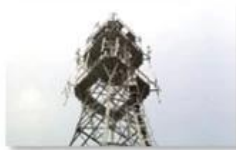
Mobile plant maintenance
