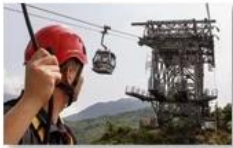
Cable car maintenance
