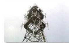
Mobile plant maintenance
