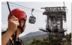
Cable car maintenance
