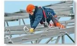
Work at height
