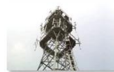
Mobile plant maintenance
