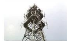
Mobile plant maintenance
