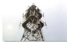
Mobile plant maintenance
