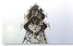
Mobile plant maintenance
