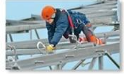
Work at height
