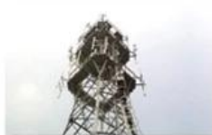
Mobile plant maintenance
