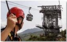
Cable car maintenance
