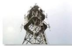
Mobile plant maintenance
