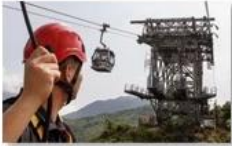
Cable car maintenance
